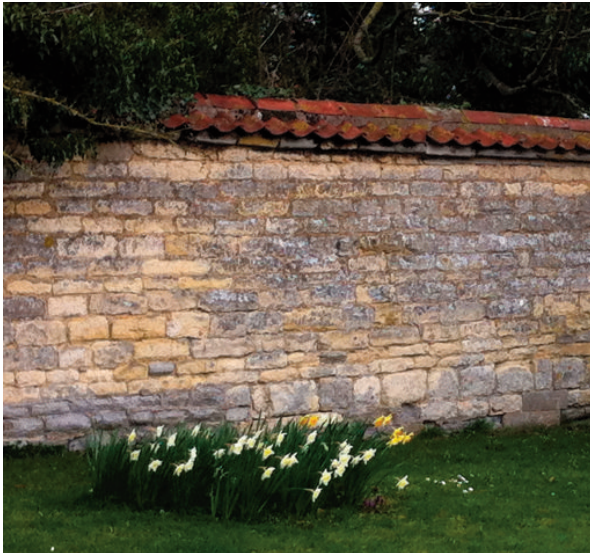
Limestone wall with pantile coping
